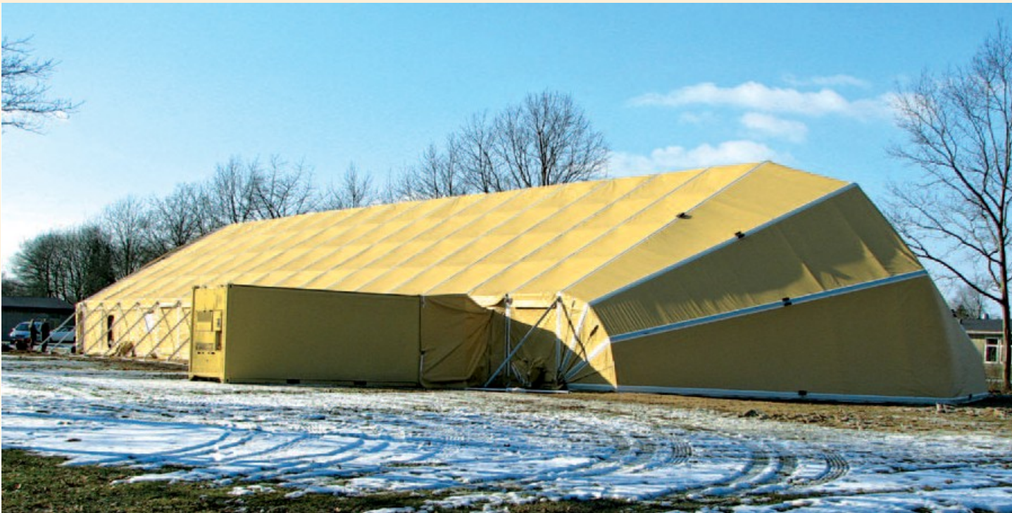
Hangar Tent with electrically driven gable and docked workshop container
