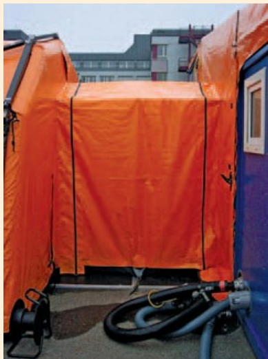
Sluice connection Tent – Container
