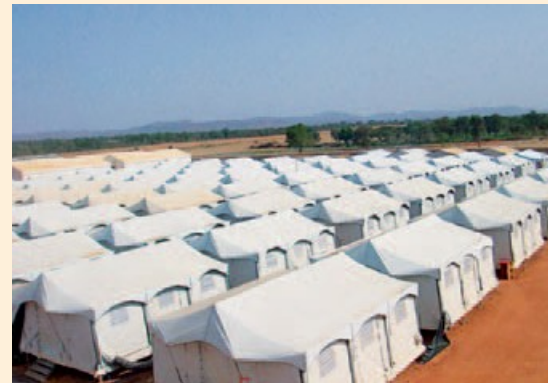
Sun roofs mounted to the Multi Purpose Tents Type EHZ II
