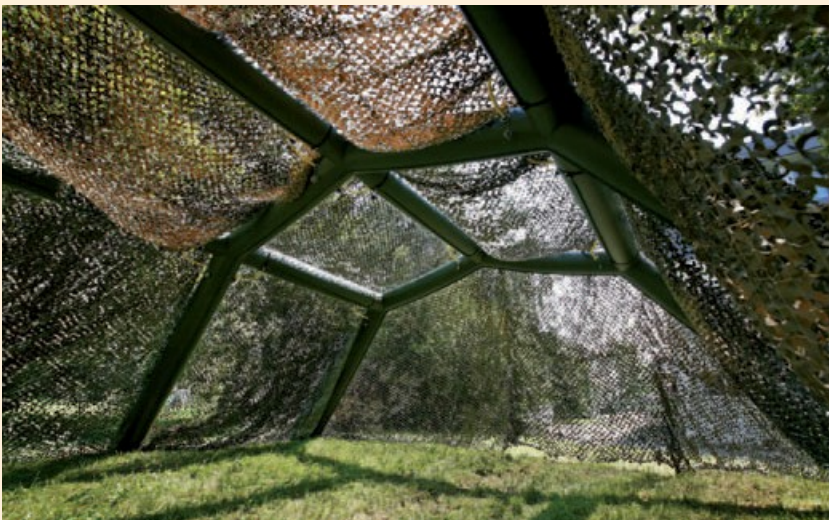
Inflatable supporting structure with camouflage nets to disguise vehicles
