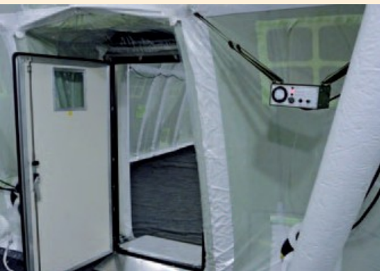
Interior view of a pressure-controlled passage
