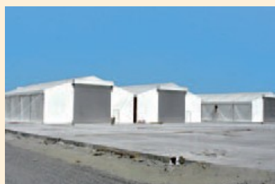
Storage Tents with rolling shutter gates in Afghanistan
